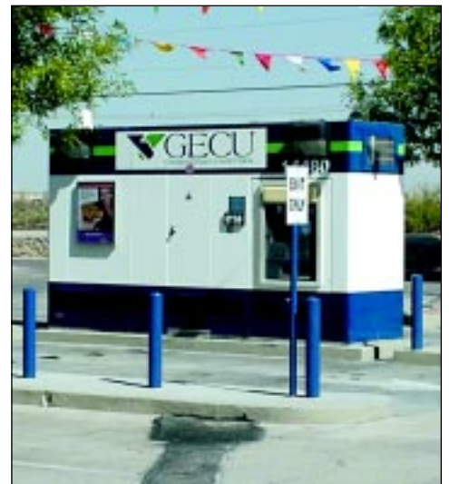
Government Employees Credit Union has installed a stand alone ATM in Horizon.
