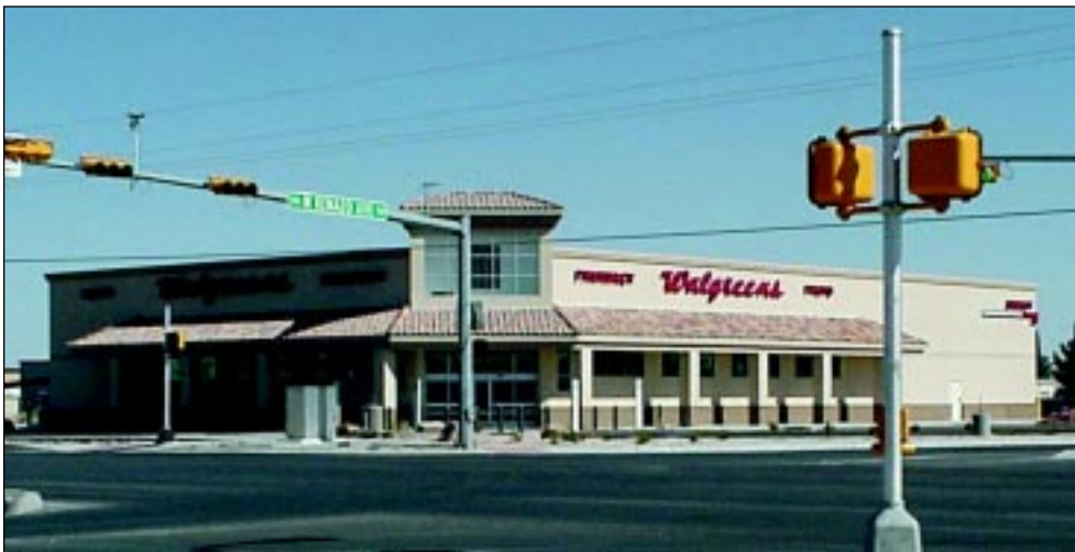
Construction is moving swiftly on this Walgreens. It is slated to open by Thanksgiving of this year.
