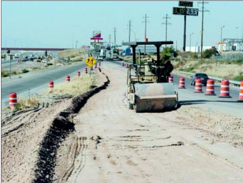
Construction of one of the new exit ramps is under way.
